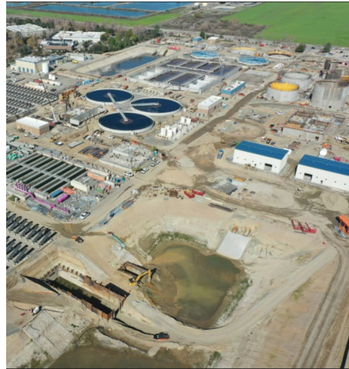
RP-5 during construction
